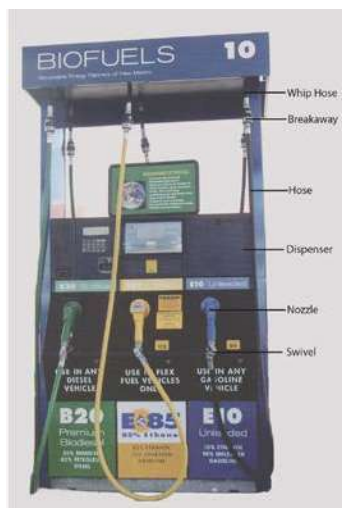
Figure 5. Aboveground equipment (NREL 13531)
